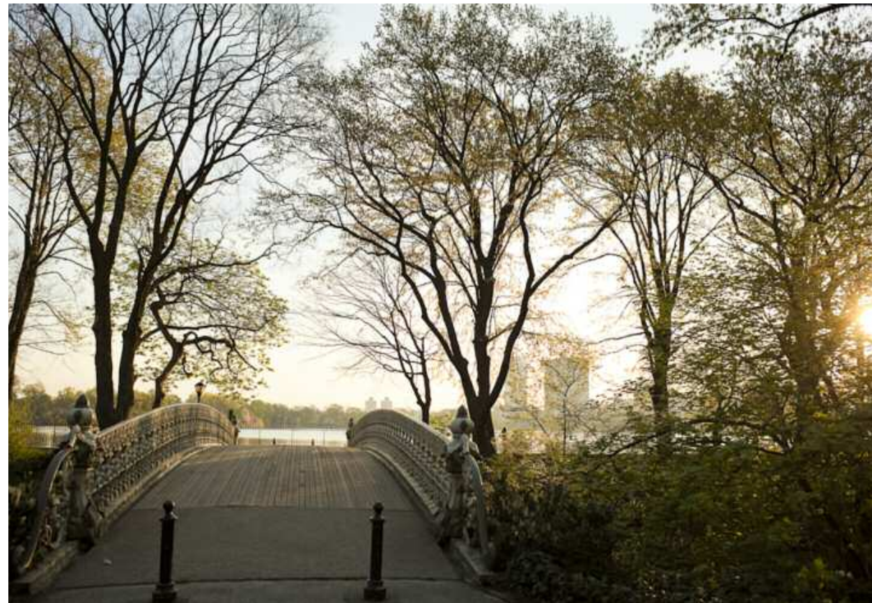
PHOTOGRAPH: CENTRAL PARK, 86TH STREET BRIDGE
